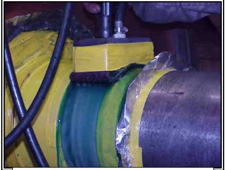
Using a flow through anode nickel plating is in process.
